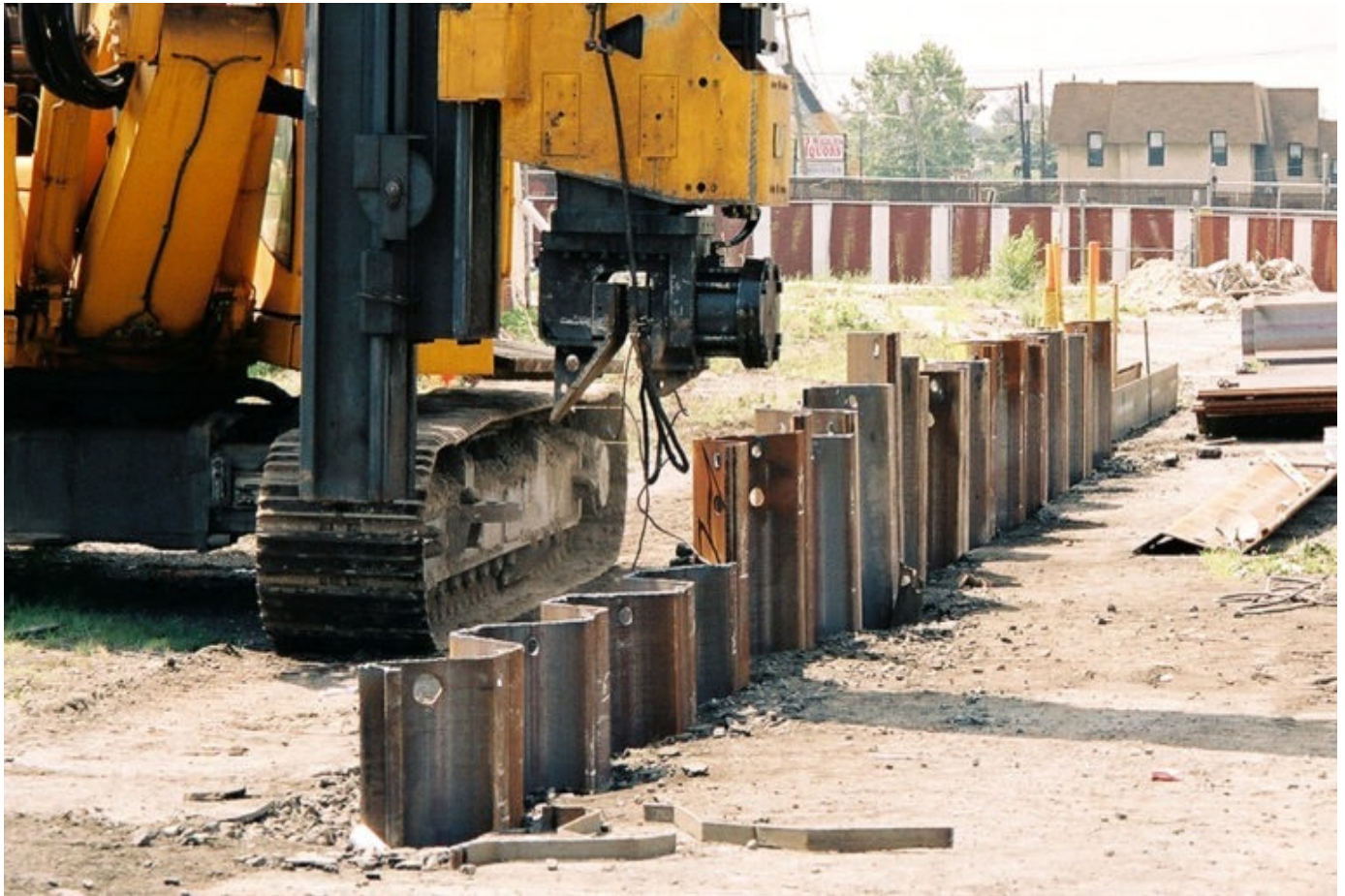
Sheet pile installation
