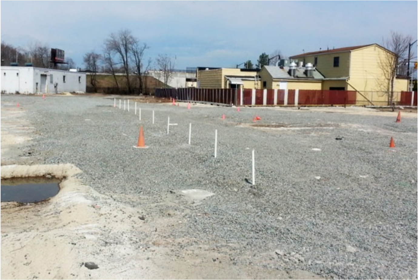
Site prior to redevelopment
