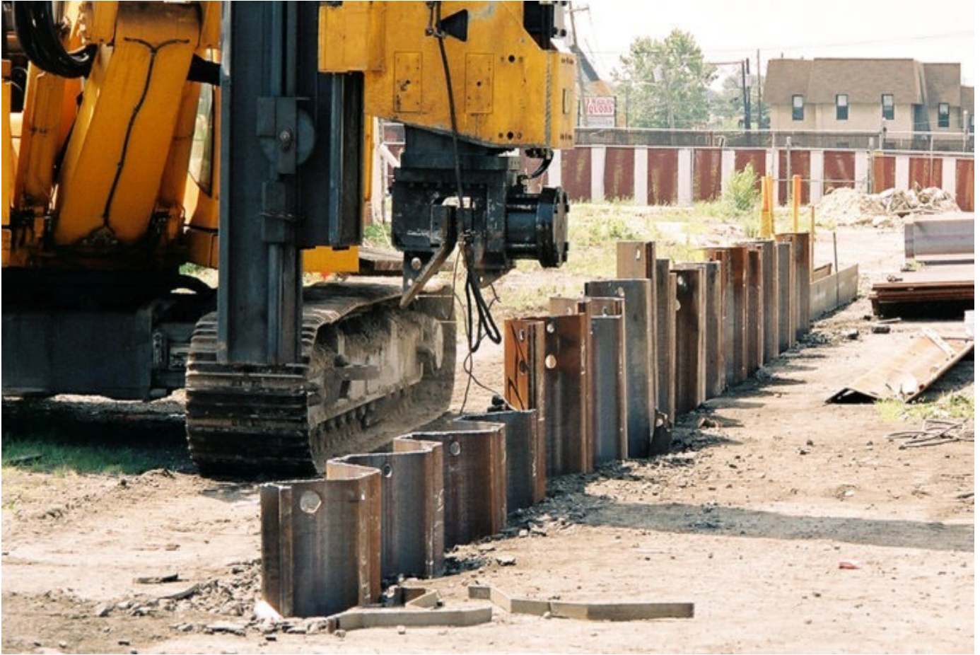
Sheet pile installation
