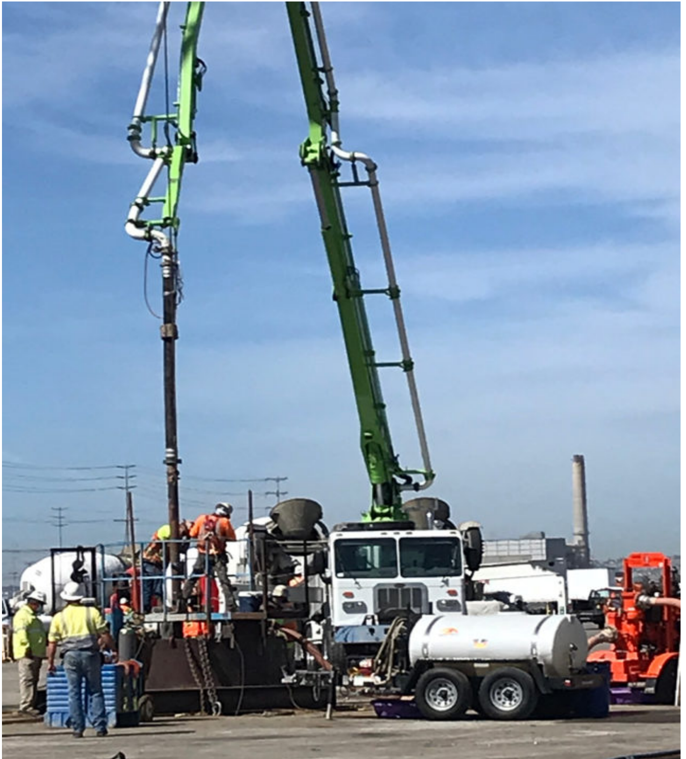
Pouring concrete to secure the rebar in place within the foundations
