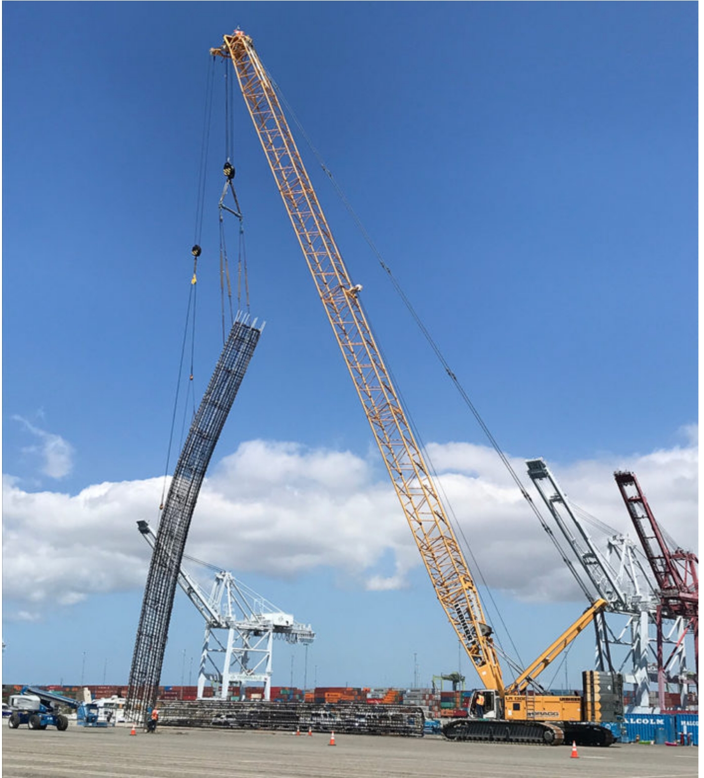
Installing rebar into the hole to reinforce the foundations
