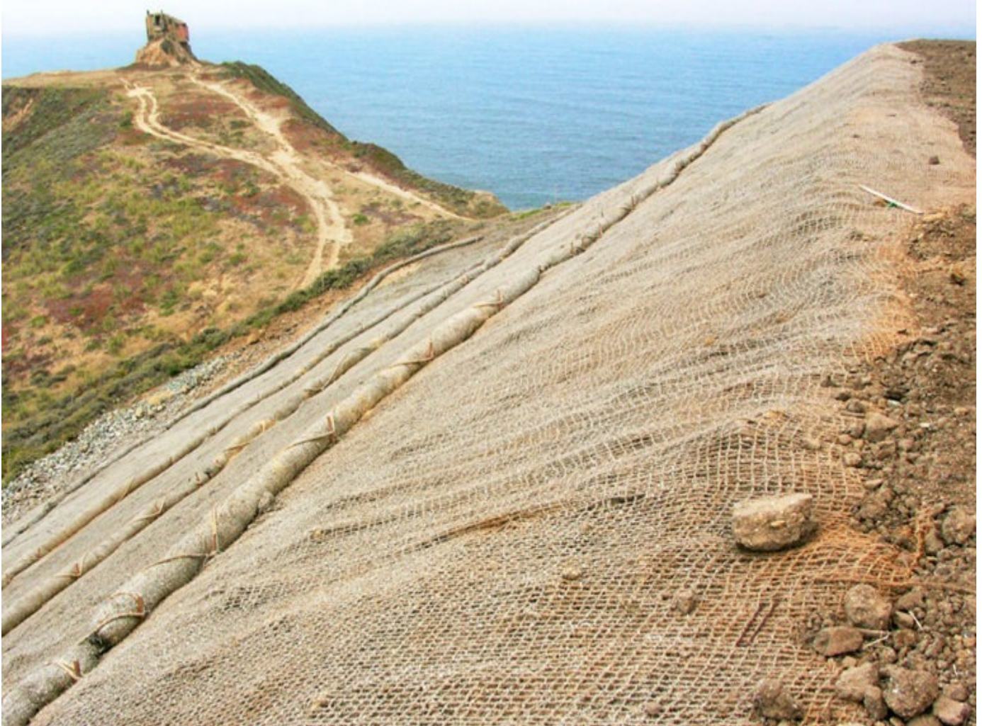
Jute netting on hillside
