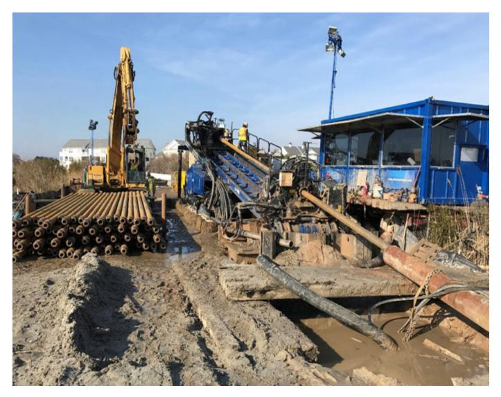
Optimal selection of an HDD landfall location requires integration of onshore, nearshore, and offshore subsurface data to develop a ground 'model' of the local conditions. When you are deciding on the location of the interface between the buried portion of the subsea cable and the HDD corridor, consider the tensile strength of the subsea cable, as well as how close to shore the cable laying vessel can get.
