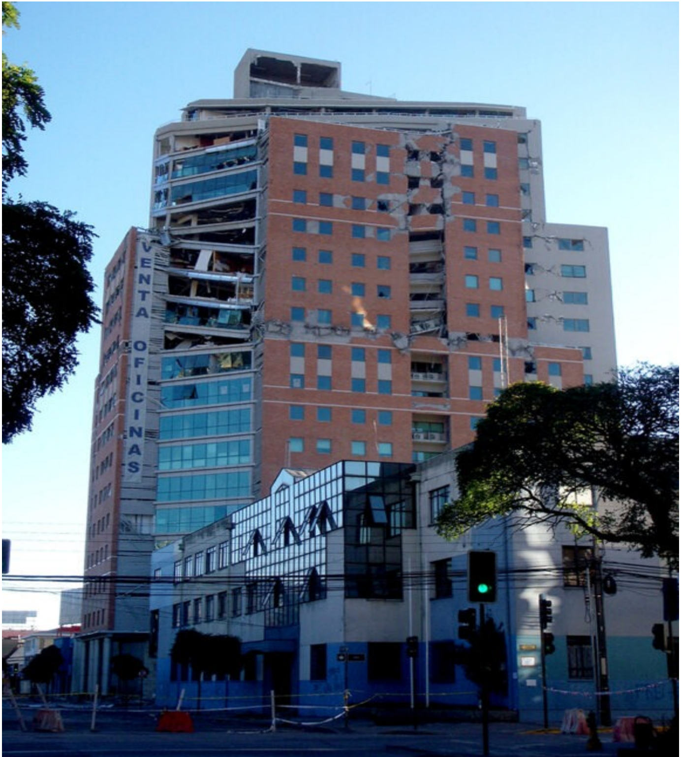
Earthquake-damaged new construction in Concepcion, Chile
