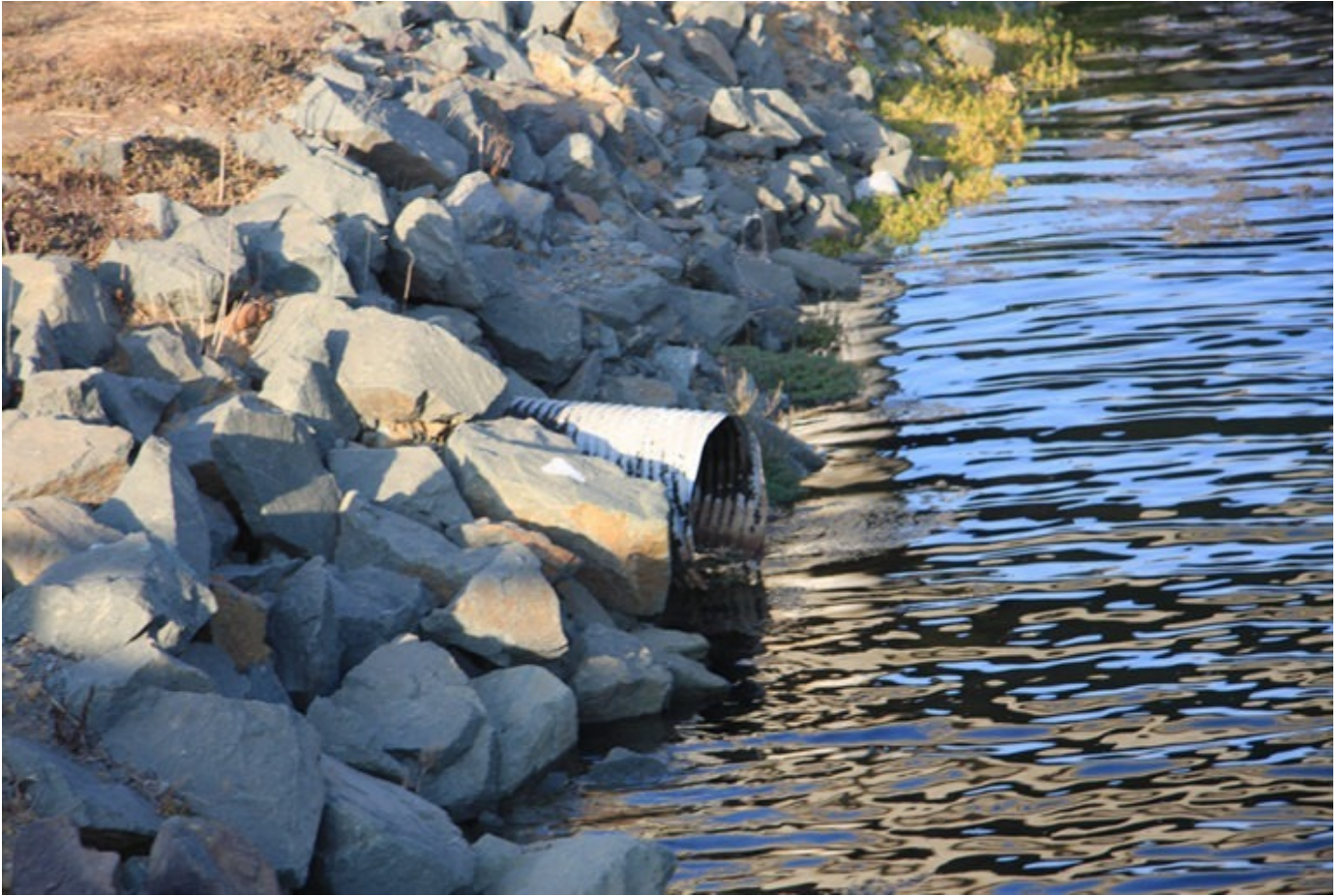
Stormwater outfall
