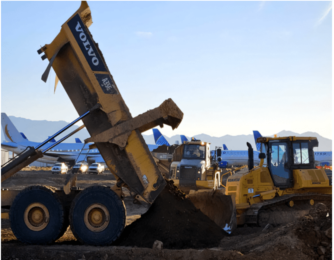
Haley & Aldrich's construction team at the Kingman project site
